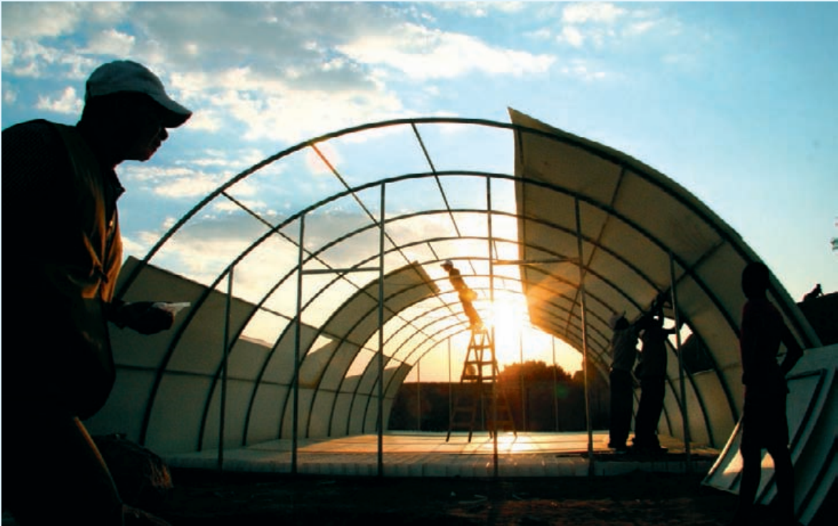
Seven new classrooms were built using fortified plastic sheets over light steel frames, one classroom for each grade. The materials came from Taiwan.
