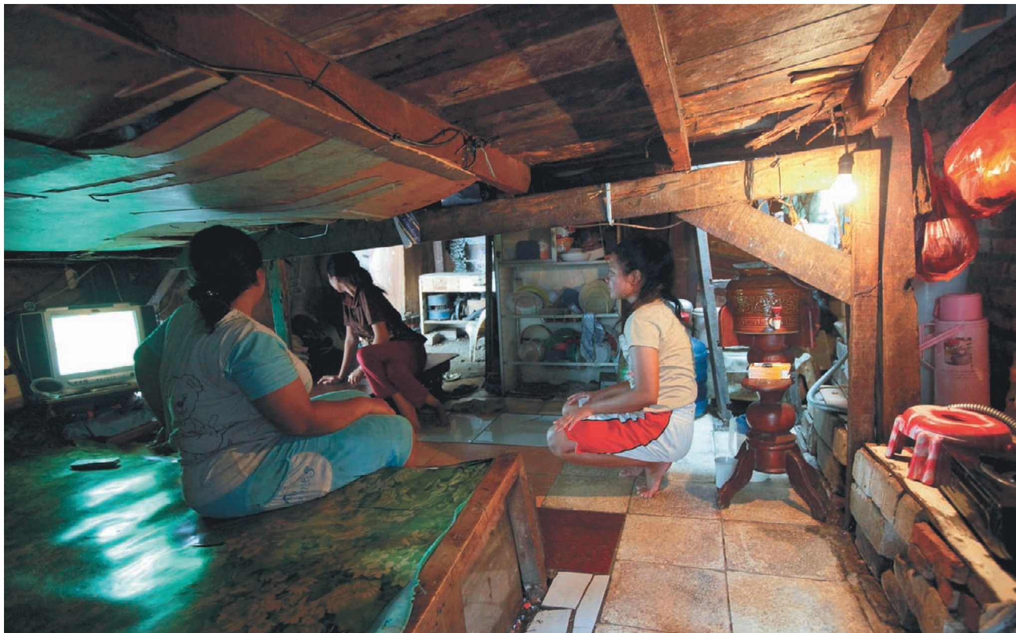
This was one of the houses selected to be replaced in a Tzu Chi home replacement project in West Pademangan. The disintegrating floor of the second story overhead indicated a dangerous situation. These people lived on the first floor and did not even have room to stand up. With not enough headroom, residents either sat or squatted in the restricted space.
