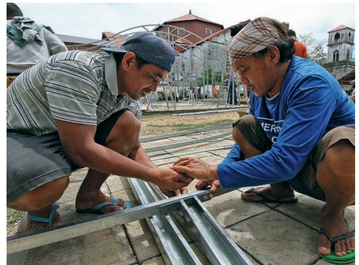
Patricio Teneza, left, works with another volunteer to assemble the frame of a prefabricated classroom.
