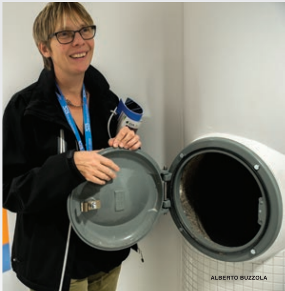
An indoor waste inlet accepts color-coded bags containing sorted garbage.
