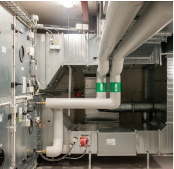
Even air is recycled. An air filter, left, extracts thermal energy from exhaust. The recovered energy is then used to heat inflowing air, right.
