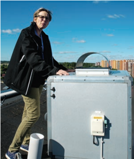
Even air is recycled. An air filter, left, extracts thermal energy from exhaust. The recovered energy is then used to heat inflowing air, right.
